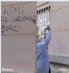
Facade cleaning - graffiti removal
