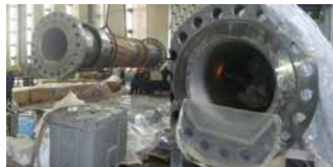
Dry ice grit blasting inside a steel pipe
